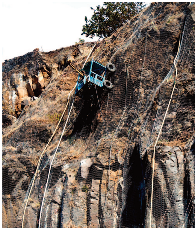
Work to stabilise the steep cliffs above Porto de Recreio da Calheta Harald Sammer
