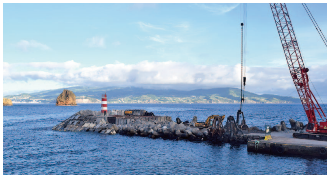
Work taking place to extend Madalena's north breakwater in June 2018. The light structure has already been moved some distance to the west, presumably to its final position. The Ilhéus da Madalena are on the left with Faial beyond. Anne Hammick
